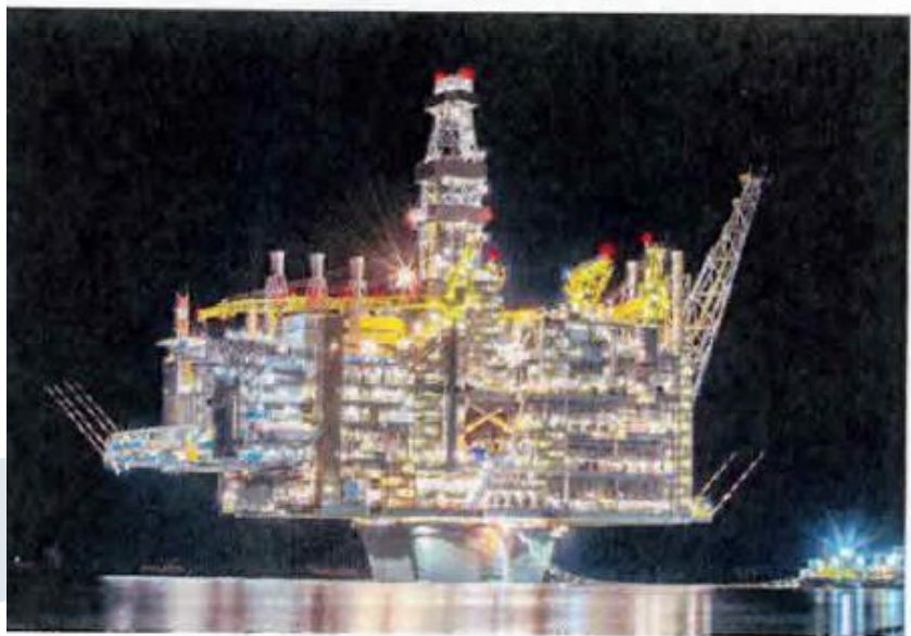
Topsides –GBS Mating complete
